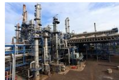
Styrene monomer plant
