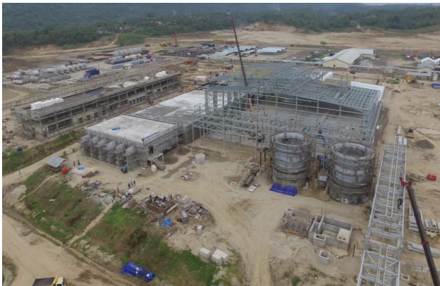
Admin, Lab & Control Room
