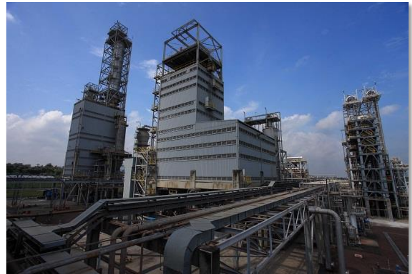
Existing PE plant in Cilegon with capacity 336 KTA with 1 train UNIPOL PE Technology 200 KTA and 1 train Showa Denko PE Technology 136 KTA
